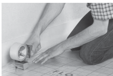
Figure 6: Sealing down the film apron
