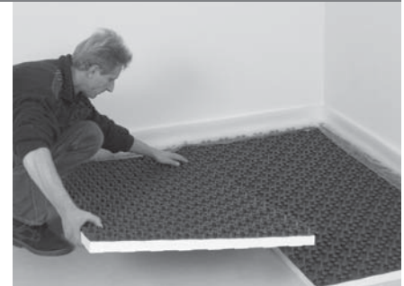
Continue laying the FLOORTEC System Preformed Plates.
