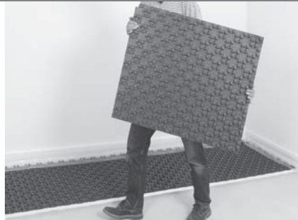
Lay the plates from left to right.
