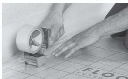
Figure 2: Sealing down the film apron
