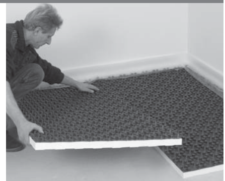
Figure 1: Installation of system elements
