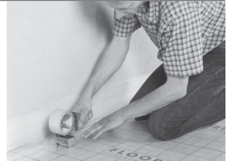
Seal the edge insulation strips using adhesive tape (if a self-levelling screed is to be applied)
