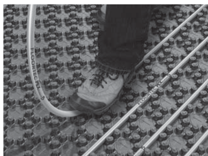
The plates can be laid quickly and cleanly, using the overlapping technique.
