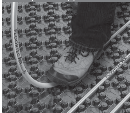
Fig. 1: Laying of Pe-Xcellent 5 underfloor heating pipe
