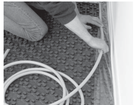
Figure 2: Fixing the additional strip of film
