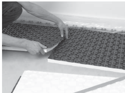
The plates can be laid quickly and cleanly, using the overlapping technique.
